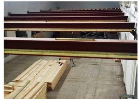
The steel beams are now in place and the mezzanine floor has been constructed which will allow the new floors to be laid shortly.
